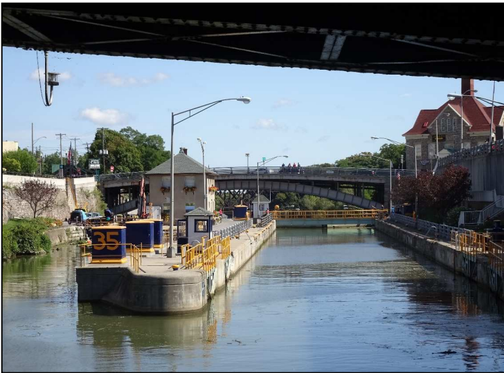
Approaching a lock
