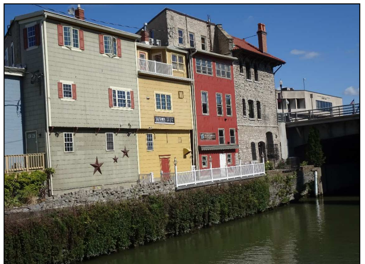
Not-so-modern home construction
